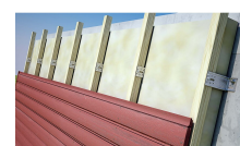
Cladding installation
