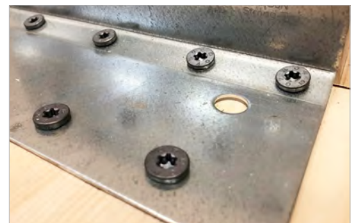
SSF screws fastening of AB255SSH angle bracket.
