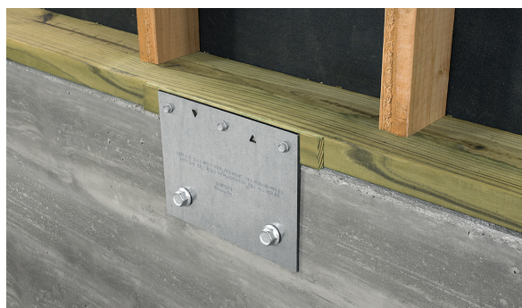
Reinforcement of the connection with the foundation
